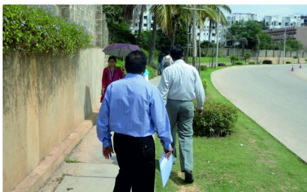
Insufficient walk way widths
