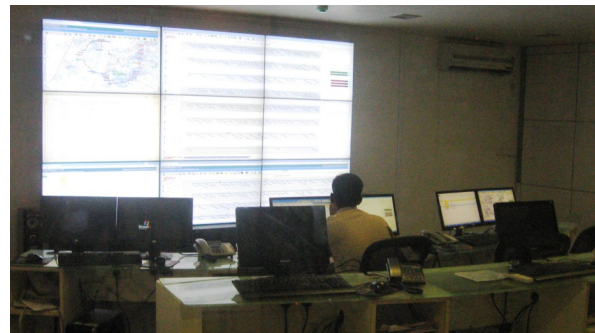
Figure 61 Janmarg BRTS Control Centre (EMBARQ India 2014)
