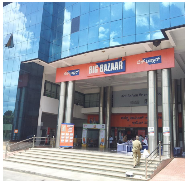
Figure 98 Commercial Development at Shantinagar TTMC (EMBARQ India 2014)
