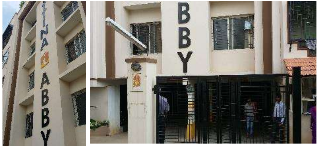
Entrance/Exit Gate at Ittina Abby, Leading Directly to Basement Parking Area
