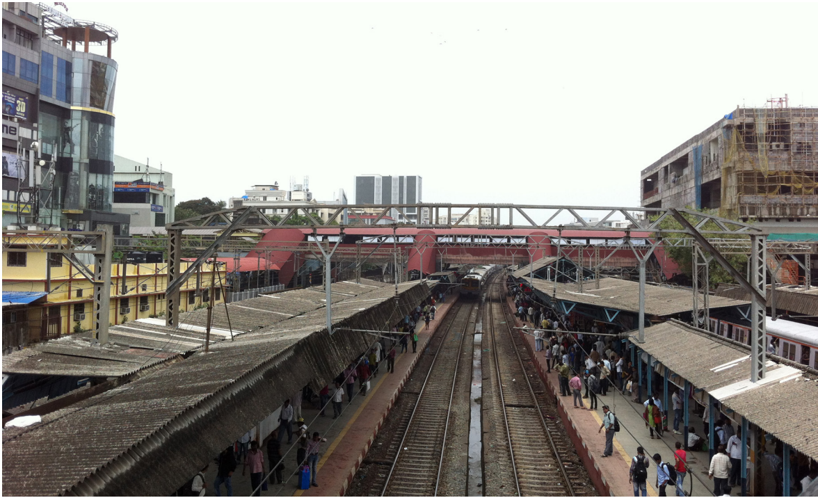
Figure 10: Image of Ghatkopar Station, Mumbai; Source: EMBARQ India
