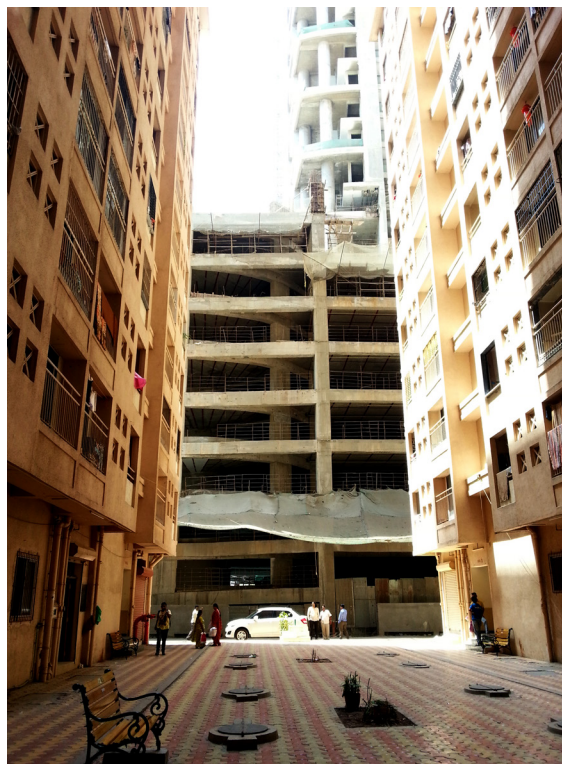
Figure 37: Development near Curry Road Station with 10 floors of parking; Source: EMBARQ India
