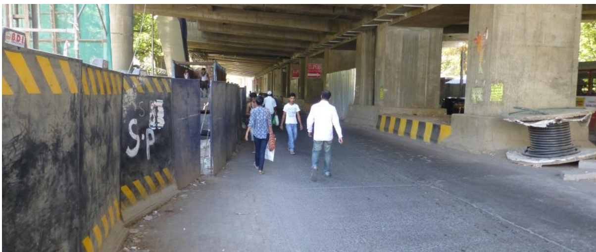
Figure 6: During construction pedestrians are forced out in the vehicle lanes
