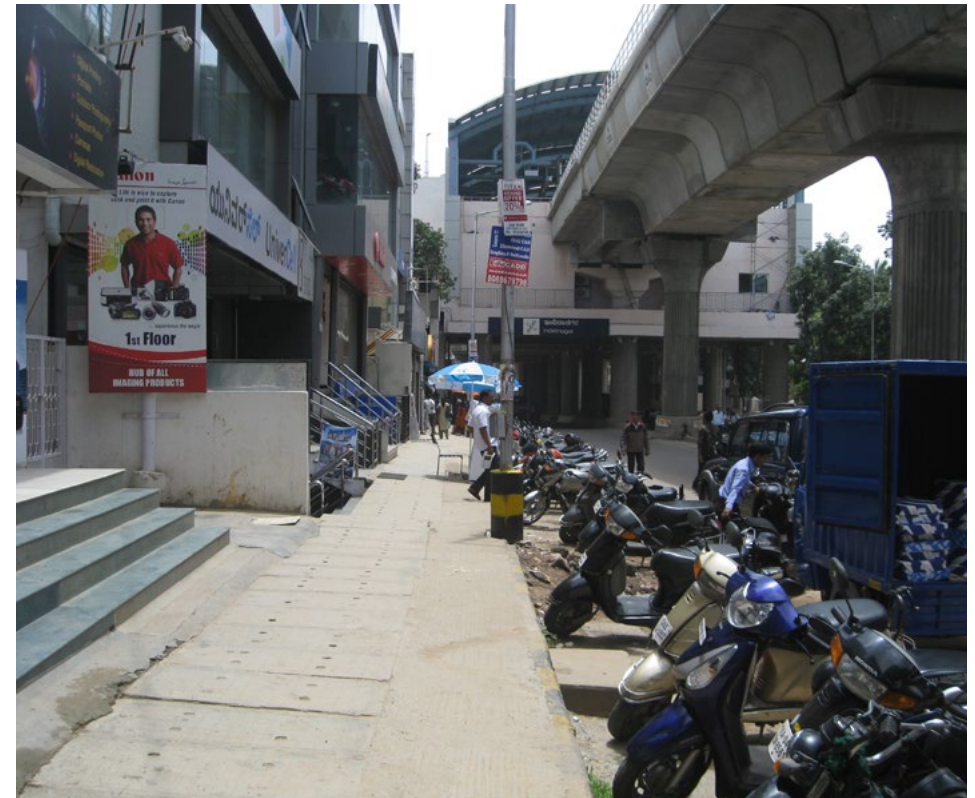
Retail activities and street use in the primary station area of the Indiranagar Metro Station
