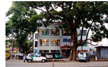
Retail on CMH Road
